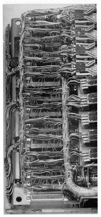
At left is a picture of components in part of the logical section of a computer made by Litton Industries, Beverly Hills, Calif. It shows wiring cables, sockets for plug-in circuit boards, nine relays (at the right), and other components. (Figure 15)
