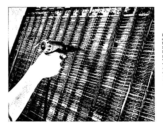
Figure 2 — Here is a maze of circuitry that goes into the logic panels of the new Bendix Corp. G-20 computer. It is wire-wrapped with this pistol-like device. Intricate wrapping and positioning of wires is handled quickly and efficiently with the powerdriven tool. Ten panels like this go into every central processor of the computer to make up the arithmetical and logical circuitry.
