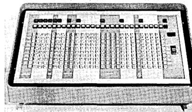
the columns where data must be entered and go out when data is entered. Automatic characters can be preprogrammed and punched at the beginning and end of each block of tape. (For more information, designate #57 on the Readers Service Card.)
