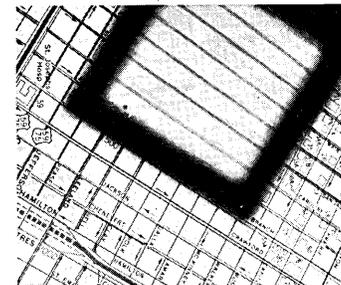
The front cover picture shows an experimental, computer-produced filter placed over a street map of Houston, Texas. The filter reveals hidden patterns in photos, charts, and other graphic material; and could be used by aerial photo analysts, seismologists, medical researchers, and quality control engineers to recognize graphic patterns that might not otherwise be detected. For more information, see page 50.
