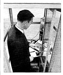
The handset of the telephone fits into the terminal's acoustic coupler, which transmits the user's signals; the computer's reply is heart over the terminal's built-in speaker, or through an earphone. The IBM 2721 has 60 keys, 26 letters, 10 numerals and 24 special characters and controls. These can be adapted for specific applications with the use of plastic keyboard overlays. To prevent unauthorized access to data stored in the computer, each 2721 can be assigned an identification code.
