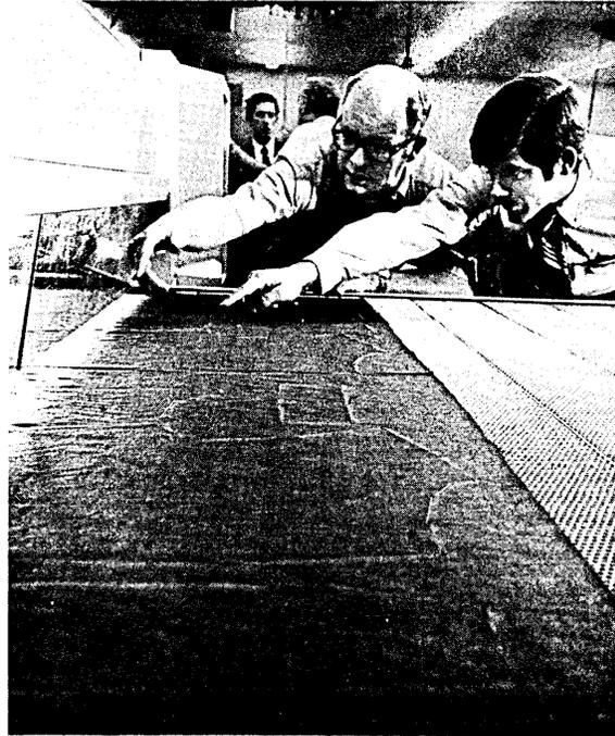
This machine, now in commercial production, consists basically of two identical crossarm positioning devices controlled by a computer which has stored preprogrammed cutting instructions for many patterns and styles, and a conveyor for moving the material from its bolt to a position directly beneath the cutting beam. The computer turns on the laser beam (not the laser itself), which then cuts (vaporizes, really) the cloth in highly complex patterns, the cut being no wider than a single thread!
