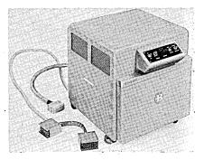
desk-size digital computer from information in punched cards. Cable-connected to the computer for simple removal and hookup, the unit is used in conjunction with modified versions of standard card keypunches. Positioning an automatic-to-manual switch allows the operator to choose whether data or instructions will be read directly from punched cards or taken from the keypunch's keyboard. Instructions entered manually from the keypunch can be simultaneously punched into cards, allowing the pro-
