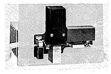
of its features – character reading speeds up to 1,000 characters per second, simple in-line threading, three millisecond starting time, stops on STOP character (0.2 millisecond) and will read next character after start, photo diode head reads any tape, ambient temperature up to 125° F with 10,000 hour life and it is not affected by temperature changes. For information write POTTER INSTRU-MENT CO., INC., Sunnyside Blvd., Plainview, L. I., N. Y., or use card.
