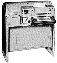
words-per-minute. The unit can also send and receive page copy on message paper or multi-part business forms, accommodate tape as a by product of both transmission and reception and provide a built-in control system for remote apparatus. Measurements: 39 in. high, 6 in. wide,  $18\frac{1}{2}$ in. deep with a keyboard projection of  $4\frac{1}{4}$  in. For information write TELE-TYPE CORP., Dept. SP-1, 4100 Fullerton, Chicago 39, Ill. or use card.
