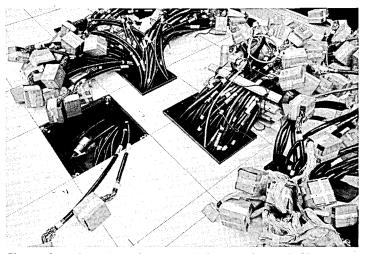
Unusual conditions can be met with floating floors. Cable cutouts can be located at any place required. The raised edges prevent casters from dropping into cable opening when moving machines.
