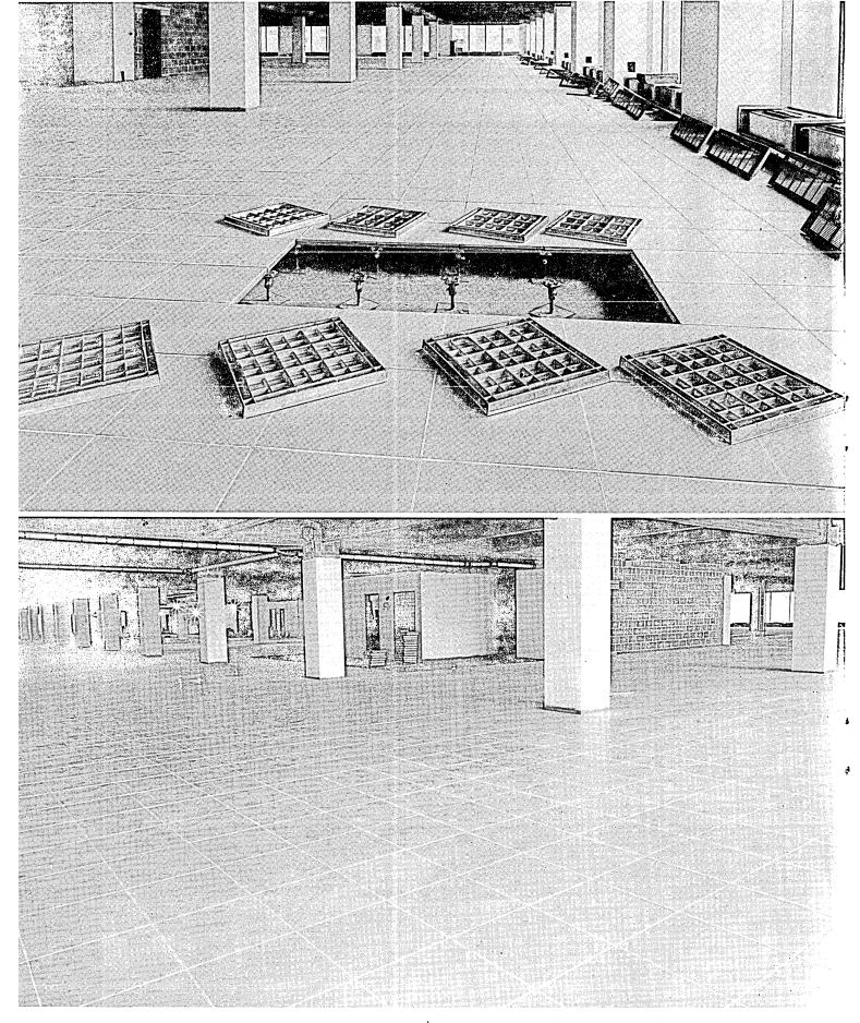
Largest floating floors installation in the world—over 150,000 sq. ft. located in New York City. This job is designed with floating floors nonconductive lip, available in any color. Safety factor on floor is 4,000 pounds concentrated load. See test photograph at bottom of next page. a floating floor is...
