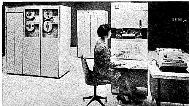
magnetic tape units, cabinets containing line termination units, level converters and line switches.
