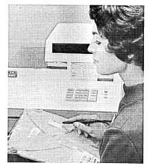
equipment. Information encoded on the labels, such as product identification and price, may also be entered manually by the operator, just as on an ordinary cash register. In addition to performing functions such as calculation of totals, taxes, and discounts, the register can also verify credit. And, of course, all of these details are recorded on tape for later processing.
