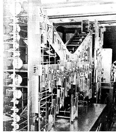
which is attached to a dial-to give a direct readout of the height of the water-and to a pen, which draws an actual curve of the tide vs. time.
