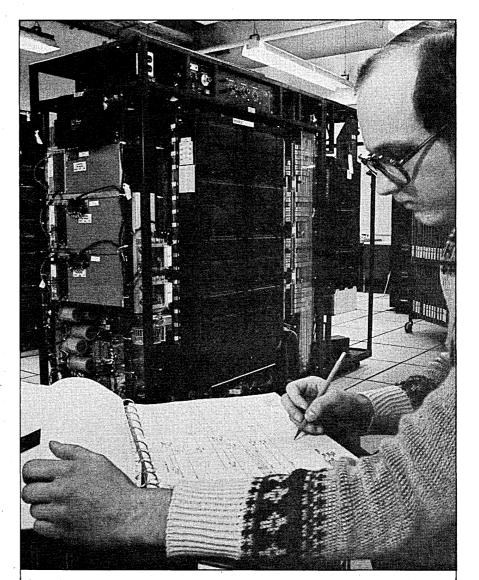
Good information on the channel directors is just now coming to the public, and this is one of the first photos to be released. Shown is frame five, which contains directors one and two (for the standard ration of channels). As can be seen, although the directors are logically "integrated" into the cpu, they are physically separate.
