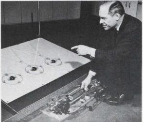
worth a thousand words, animated displays will have a major role in the show. Typical of these is the set-up that will be used to explain laser action (see illustration). Electrons are represented by cork balls and photons by an array of 324 lamps. An Actan rotating-drum memory switch, made by the Sealectro Corp. of Mamaroneck, N.Y., controls the symbolic interaction of the electrons and photons by programing the lamps and balls.
