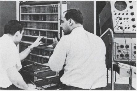
**Engineers debugging a component** of an on-line computer system under actual operating conditions at Western Union's computer research laboratory.
