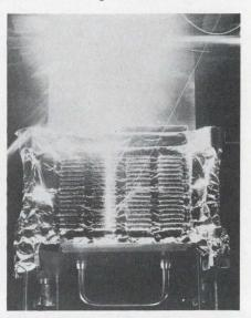
Electron beam welds a row of terminals in an IBM ferrite memory plane. The arrays move past the beam automatically on the production line.
