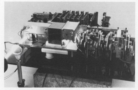
Lockheed's candidate for the Air Force's laser communications satellite system is a single-frequency system that operates continuously in a single longitudinal and transverse mode (TEM<sub>oo</sub>). The competing system by McDonnell Douglas is a mode-locked pulse device. Both systems use lithium tantalate modulators.
