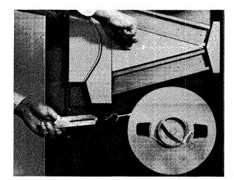
Figure 6-3 Measuring Drag Brake Torque
