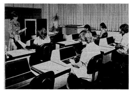
At the rear of this typical Key-Edit 50/60 work area are the processor cabinet, magnetic tape drive, supervisory console, and optional line printer.
