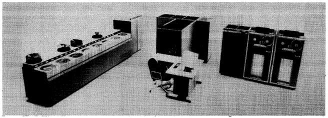
Here the Advanced System mainframe is flanked by Itel disk and tape subsystems. Itel Corporation is a major third-party lessor of IBM computer equipment and claims to be the leading independent supplier of 3330-style disk drives and monolithic add-on main memory.
