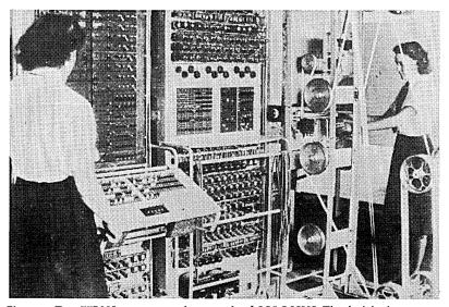
Fig. 3.2 Two WRNS operators at the controls of COLOSSUS. The deciphering process was interactive, in the sense that an operator was able to alter the sequence of trial cipher keys in the light of meaningful transliterations which might appear on the machine's printer. Full details of COLOSSUS and other wartime code-cracking machines are still secret.
