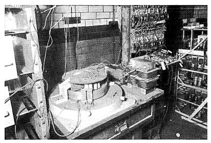
Fig. A2.1 Research on a shoe-string: the servo-synchronised magnetic drum store of the Manchester University Mark I computer in 1949. Because of its squat shape, the nickel-plated drum was referred to locally as the 'magnetic wheel'.
