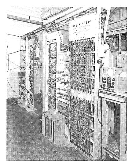
Fig. 11.2 The Theory Laboratory at Borehamwood, receiving a contract to compute trajectories, realised that the easiest and most interesting way to solve the tedious calculations was to build themselves a computer. NICHOLAS was the result. It was in parts literally home-made, and the wooden frame and consequent fire extinguisher may be seen in this photograph. NICHOLAS performed valuable service from 1952 to 1958.
