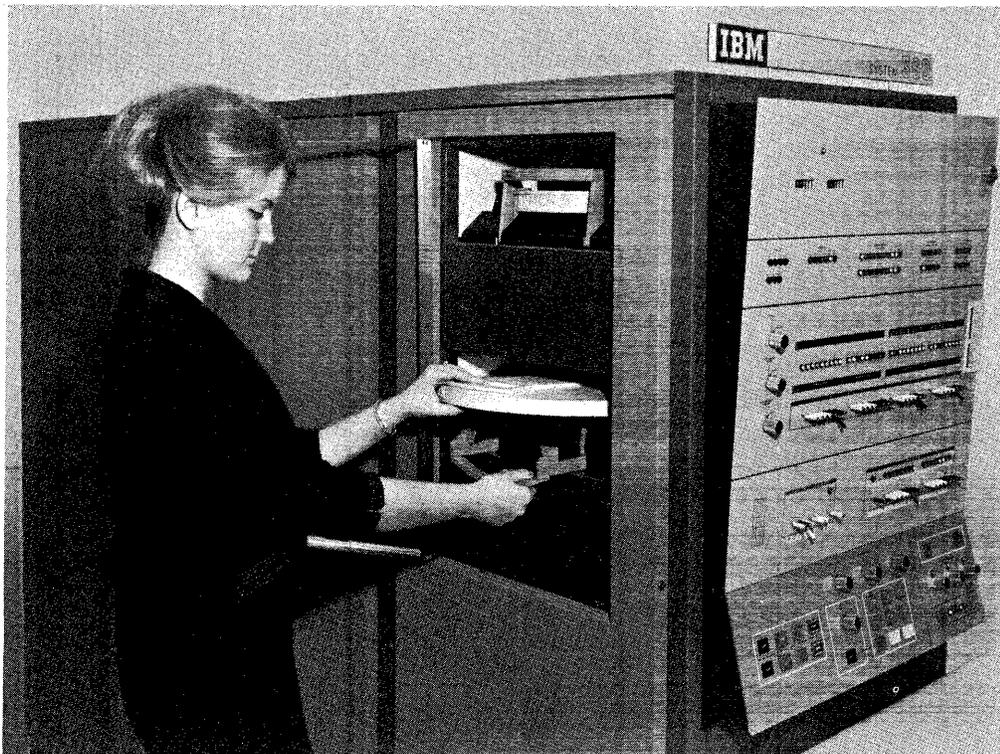
● Figure 5. Removing an IBM 2315 Disk Cartridge from a Single-Disk Storage Drive
