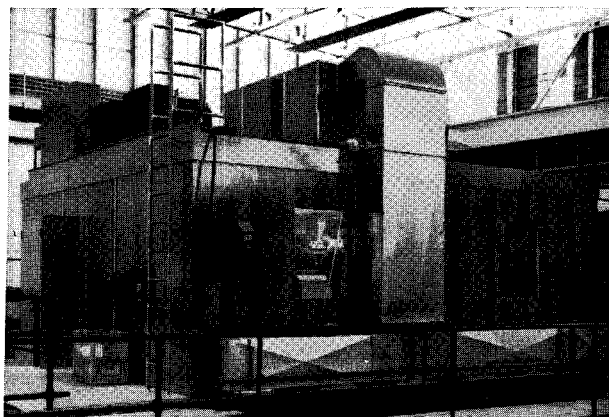
Figure 5 The installation of the IBM 360/44 in the experimental area. It can be moved easily (e.g., by a crane) in three parts: the air cooling equipment on the roof and the hut with its content in two halves.
