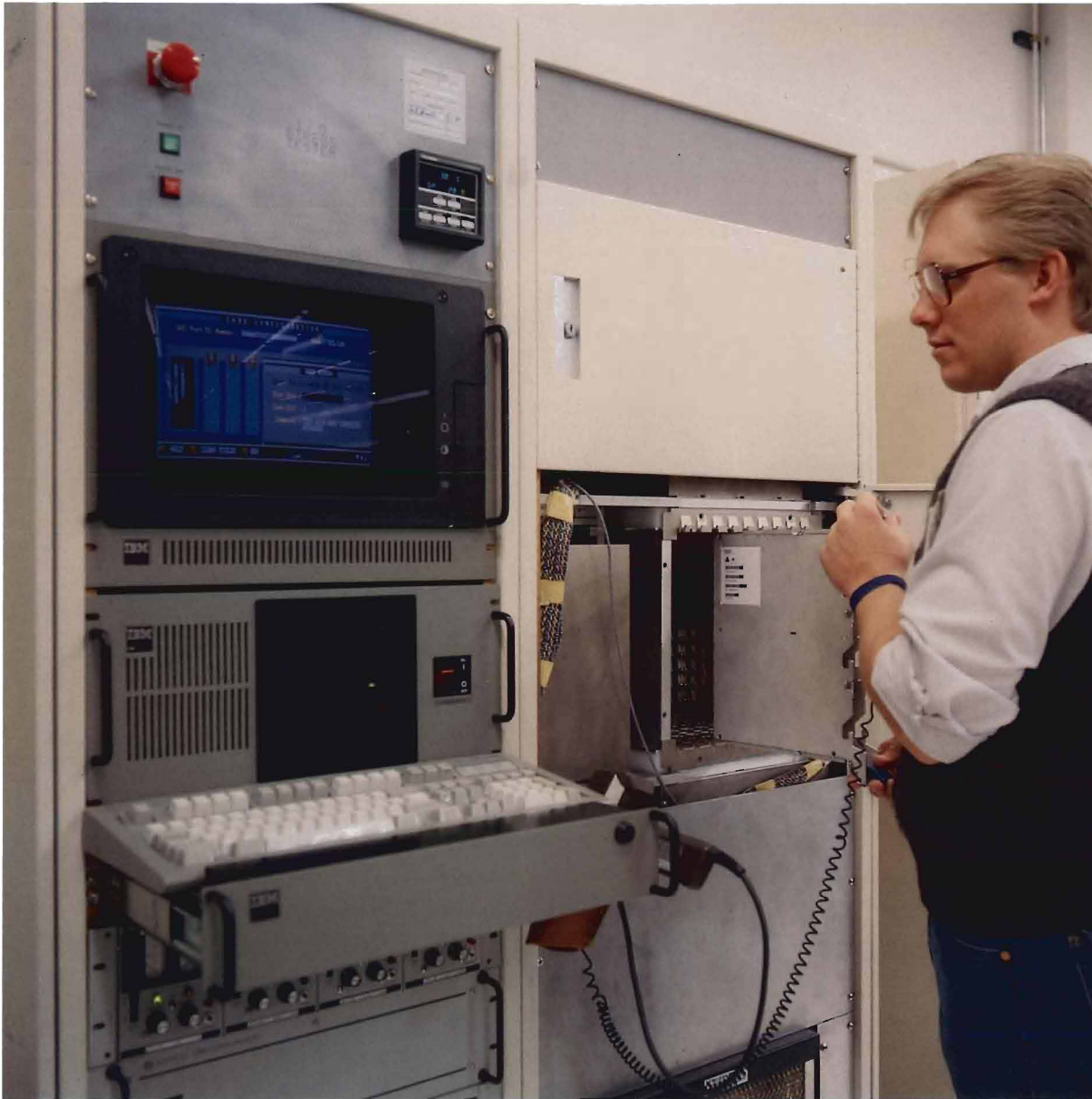
Figure 3 Logic Card Being Functionally Tested
