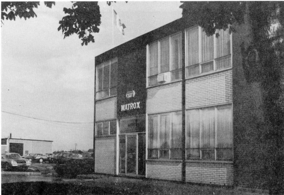
Figure 3. Matrox 22,000 square foot administration and engineering facility in Montreal, Canada.
