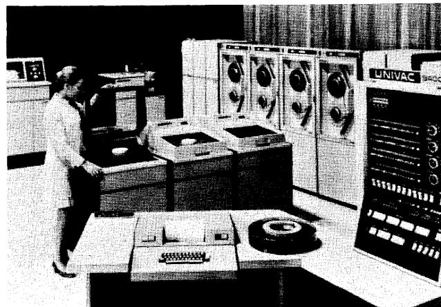
*This closeup of the 9400 console also shows three of UNIVAC's 2311-compatible 8411 Disc Drives.*
