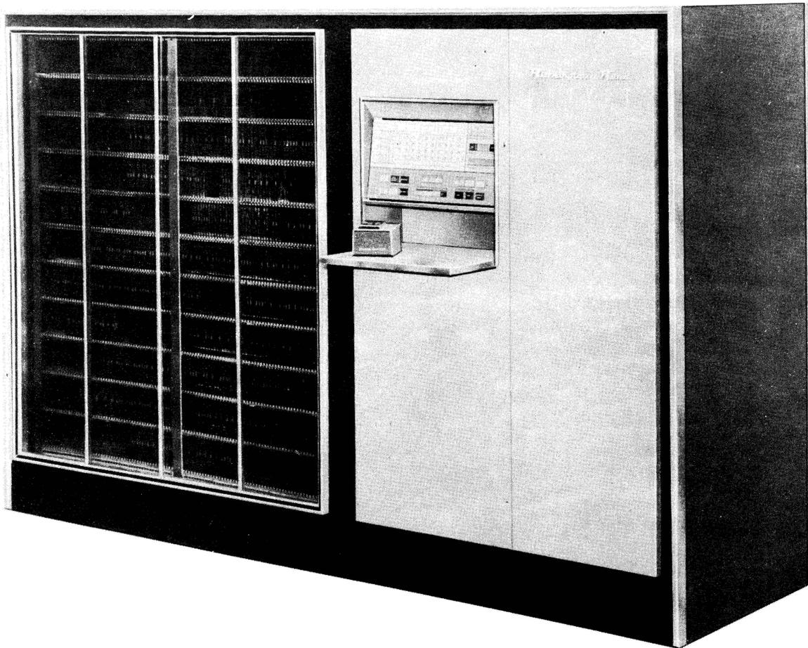
The **CENTRAL PROCESSOR** is the control center of the UNIVAC Solid-State Computer. It houses the arithmetic and logical circuitry, the data storage system, the power supply system, and the operator's panel and keyboard.
